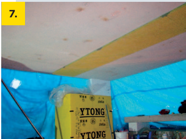
7. Installation of the first row of slabs - inspect the straightness of the row
