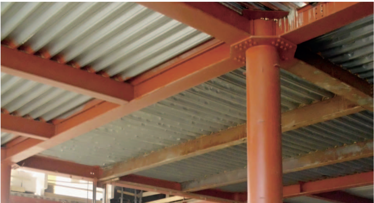
Fig. 17 If the reinforcement is placed in the trapezoidal sheet waves, a ribbed ceiling with a bearing "T-section" will be formed and therefore a statically optimal use of the height of the concrete slab will be achieved. When establishing the insulation capacity criterion I, you can consider the height h_1 or the so-called effective height of h_{\text{eff}} ; the thickness of the distribution layers h_f can also be included in I criterion in individual cases.
