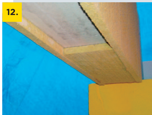
12. The flange is glued in the end
