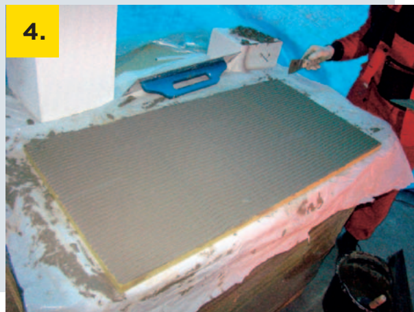
Spread the adhesive with a notched trowel over the entire surface of the slab
