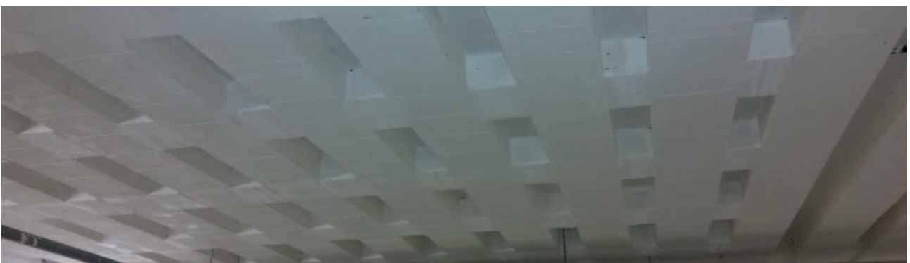
Fig. 19 Final appearance after applying white paint to the insulation surface
