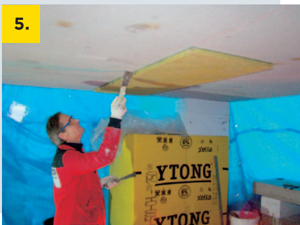
Press the first slab to the baseline and remove any excessive adhesive
