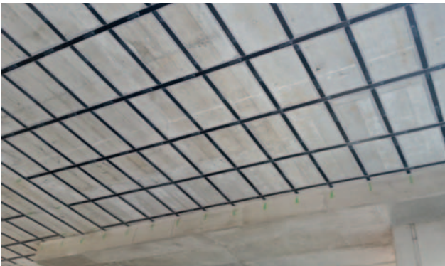
Fig. 17 Carbon fiber reinforced lamellas before fire protection
