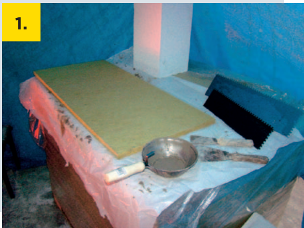
Inspect the slab and the tools used
